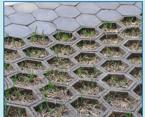
*Disconnecting impervious areas allows stormwater to infiltrate into groundwater.*
