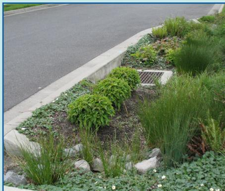
*Installing vegetated filter strips between curbs and drains can reduce pollutant loading.*
