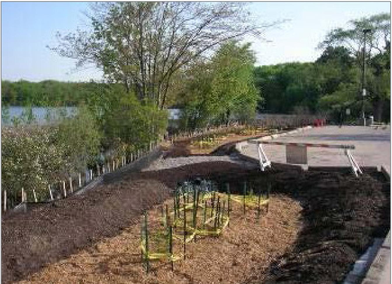
**Figure 6-2:** Adding a bioswale at edge of a parking lot
