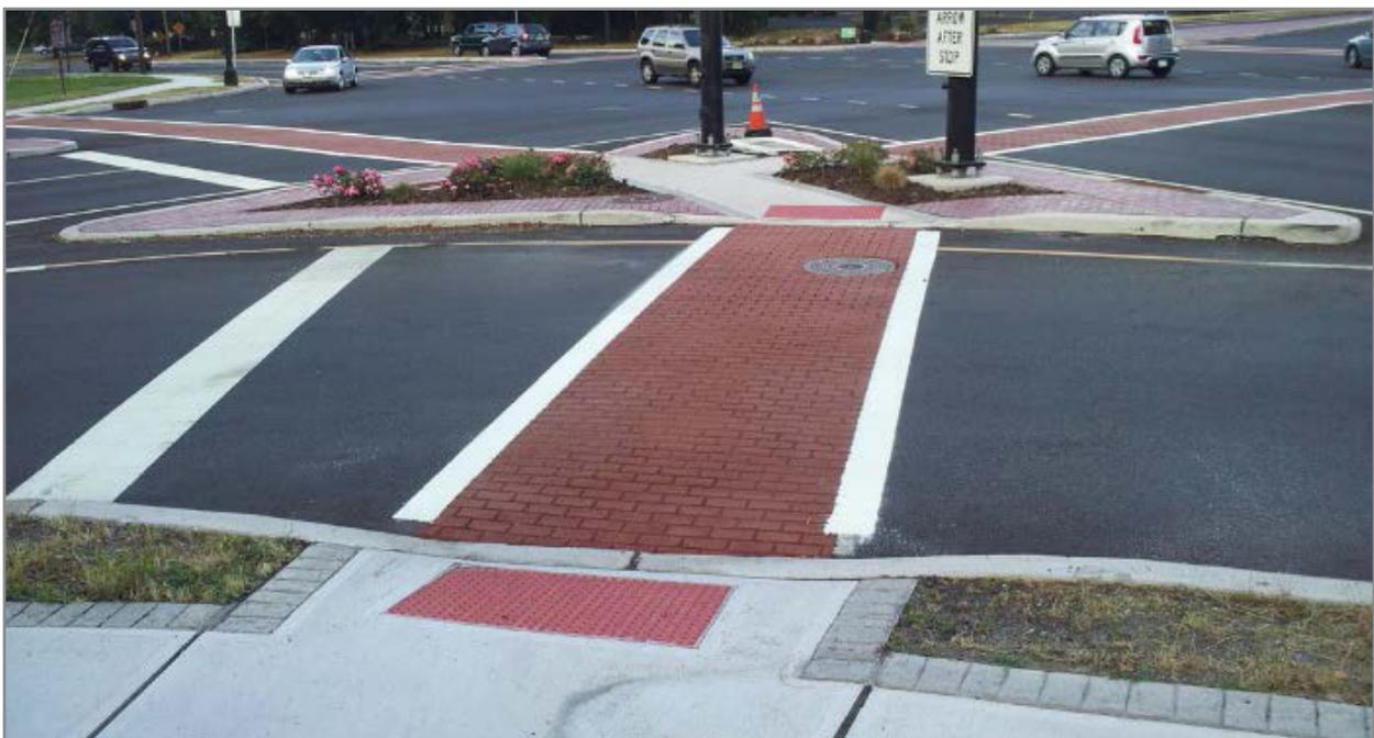
**Figure 6-12:** Pedestrian crossing constructed with pervious pavers.
