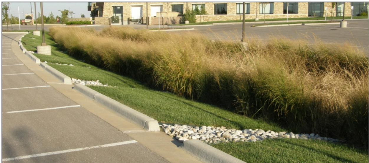
**Figure 5-12:** Picture of a bioretention facility. (Photo courtesy of David Dods)
