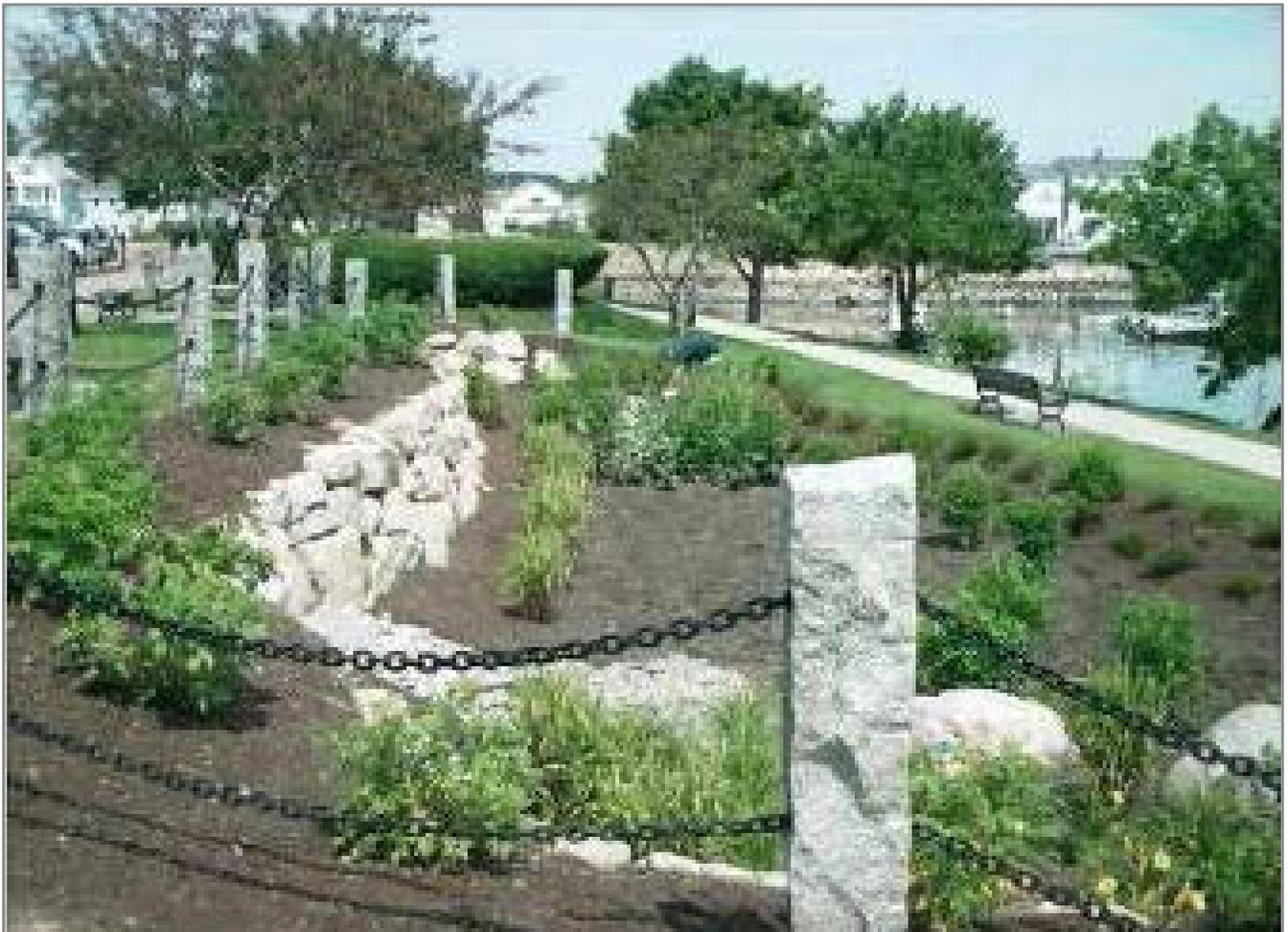
**Figure 6-1:** Adding a Bioretention basin (rain garden) in a municipal park
